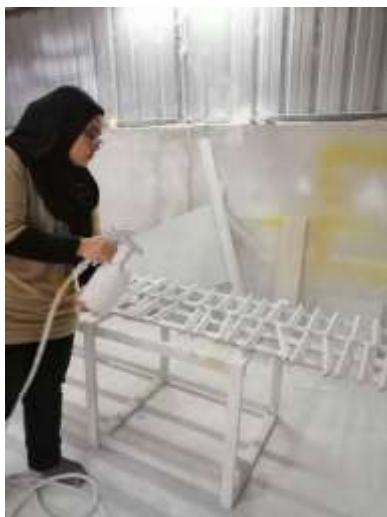
Figure 1. The coating process
