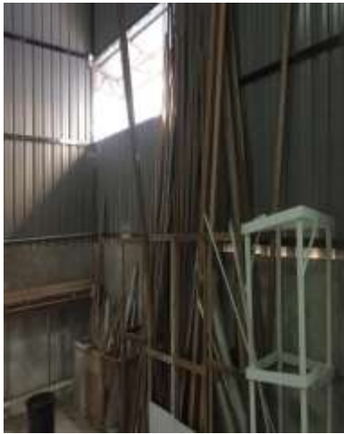
Figure 6. The area for stocking the wood panels
