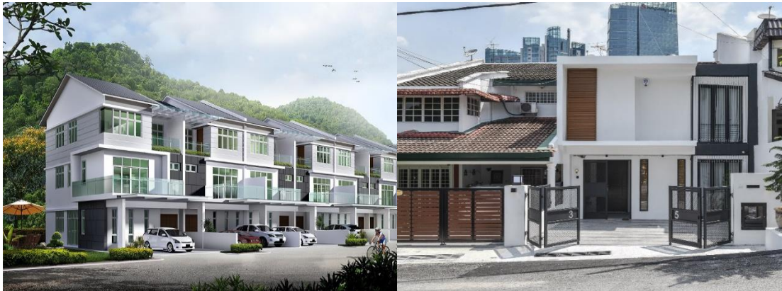
Figure 7. Pseudo-Nouveau Façade for Residential in Malaysia
