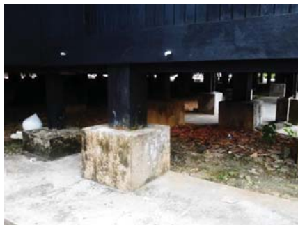
FIGURE 9. A closer view of Masjid Kg. Laut which was built on stilts.
