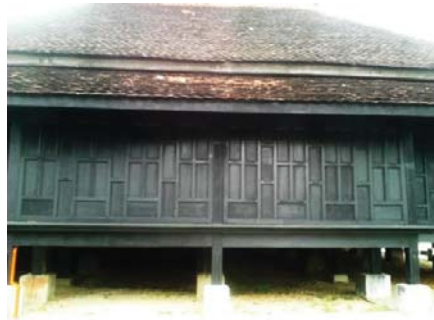
FIGURE 8. An external view of Masjid Kg. Laut which was built on stilts.
