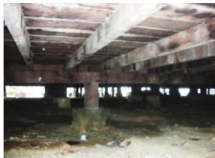
FIGURE 10. Underneath the floor (view from under) (Hassan & Nawawi, 2014).
