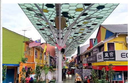
Figure 4.0: Pedestrian mall canopy
