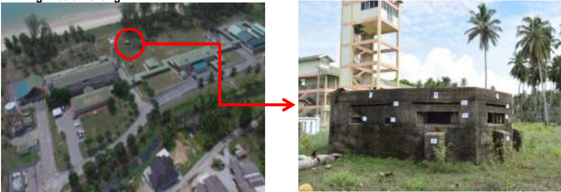
Figure 10: Location of the British pillbox at Kg Kuala Rejang, Bachok, Kelantan. Source: Field study and IOESUM (2012).
