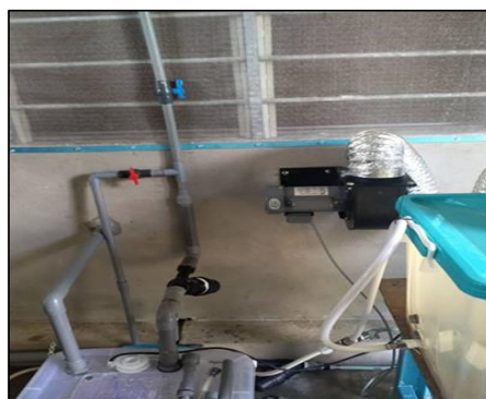
Figure 2. Installation of watering and drain system
