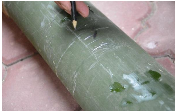
Figure 6. Marking the midpoint between the two segments
