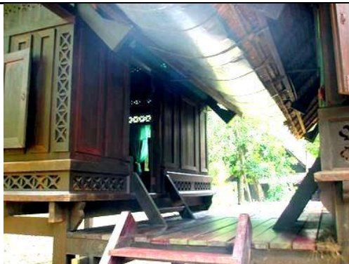
Figure 3: Gutter is made from metal sheets (Source: Utaberta et al., 2015)
