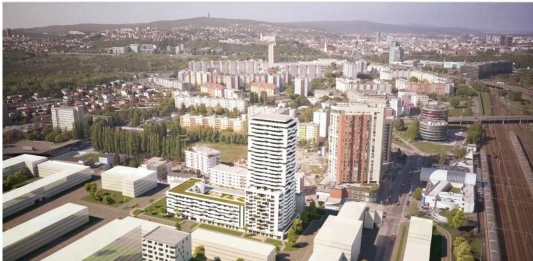
Figure 6: Visualization of Matadorka (in foreground), a multifunctional residential complex currently being built on the former Matador industrial area.
