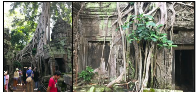
Figure 4. Domination of the plant's roots damaging the structures of Ta Prohm's temple, Cambodia.
