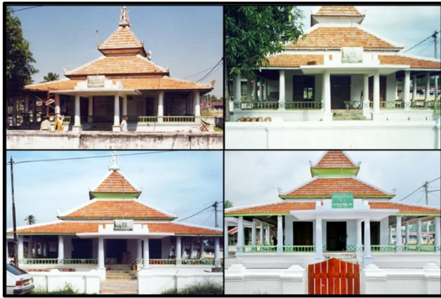
Figure 7. Conservation work in Ayer Barok mosque, Malacca showing the presence of mango tree ( Mangifera indica ) at the side of the mosque. (Source: website ntqt.com.my)
